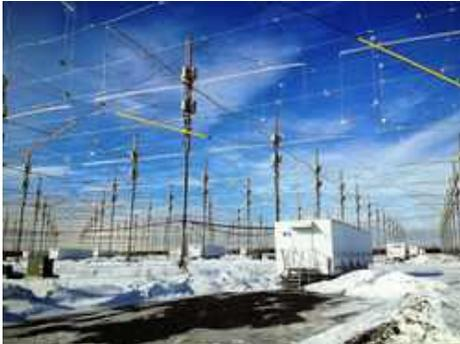
HAARP consists of multiple transmitters feeding 180 phased-arrays and is capable of producing 3.6 MW (that's megawatts) of RF. HAARP's signal is essentially aimed straight up.
